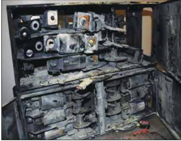
Figure 2. Arc flash on a solidly grounded system
