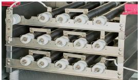
HRG systems are the safest and least expensive system available today. IEEE supports this by saying, "A safety hazard exists for solidly grounded systems from the severe flash, arc burning, and blast hazard from any phase-to-ground fault." (IEEE Std. 141-1993, The Red Book).
